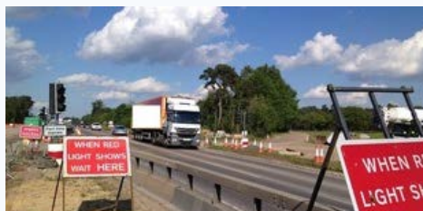
A11 dualling work to be completed in December
